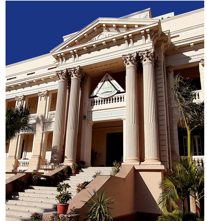
Photograph of the Heritage Administrative Building of Benha University.
